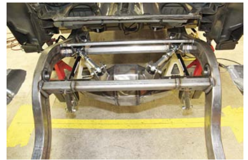
■ After aligning/squaring the back-half frame clip with the suspension assembly, it was then removed and cut to fit.
